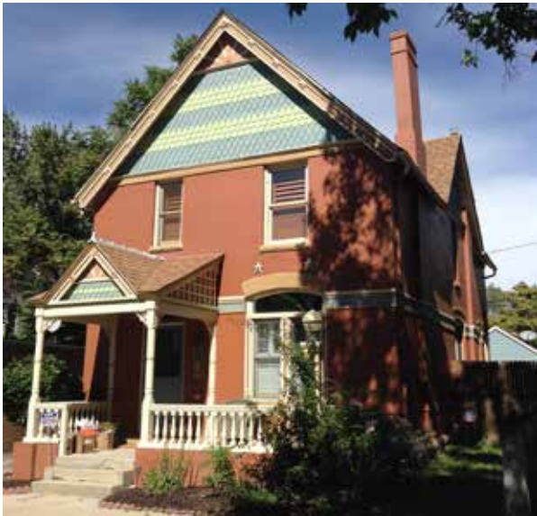
6. Typical Queen Anne development within the district. Note the forward facing gable with fish-scale shingles and decorative sunburst and barge board, the projecting front porch with cross gable roof with a matching fish scale shingles and sunburst motif, and the arched ground-floor window.
