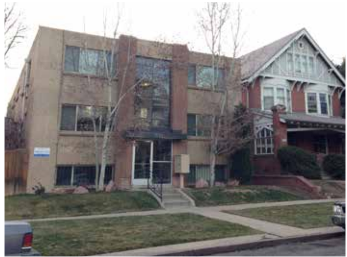
6. Mid-century apartment buildings are generally two to four stories high and have simplified forms and ornament. They usually do not have porches or balconies.
