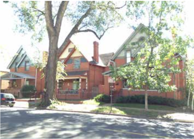
1. Street view of Queen Anne style homes within the district. Note the forward facing gables, one story porches with shed and gable roofs, the large windows, asymmetrical appearance of the front façade and overall architectural harmony of this block. Middle porch is original; two flanking porches are early 20th century additions – historic but not original.
