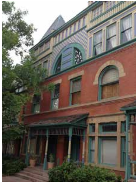
5. Queen Anne rowhouse on 21st Street. Note the historic sandstone sidewalk, brick construction with stone foundation, steeply pitched slate roof, and the one story porches with fretwork and spindle columns.
