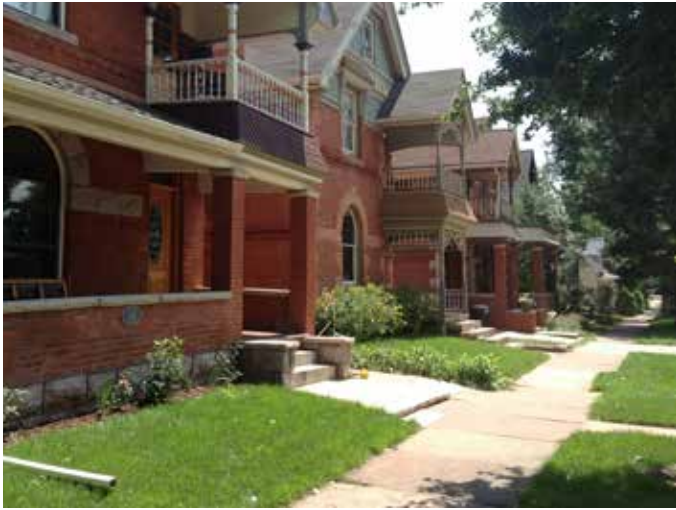
7. Streetscape within Potter Highlands. Note the historic walkways that are offset leading in a straight path to the entry door.
