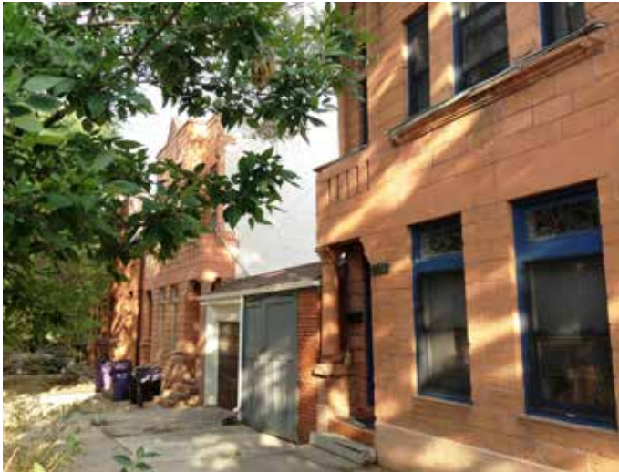
8. Stonemen's Row with accessory garages. Note the small bays, single bay opening, the flat roof and the brick construction. In this portion of the district, the structure align with the sidewalk, eliminating walkways.
