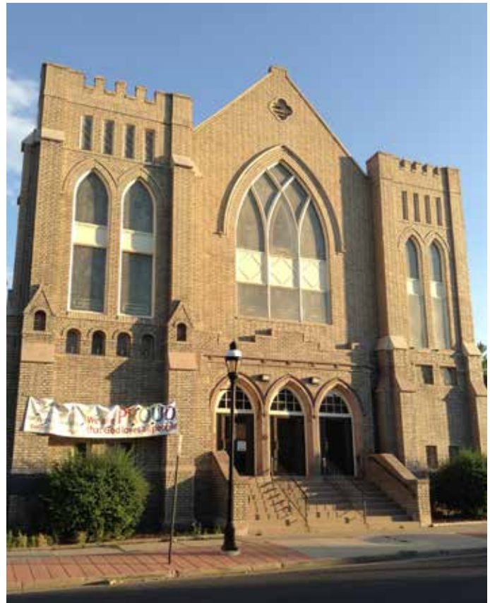
6. Gothic Revival Church. Note the arched windows with tracery, the crenellated side towers and the "castle-like" appearance of this structure.
