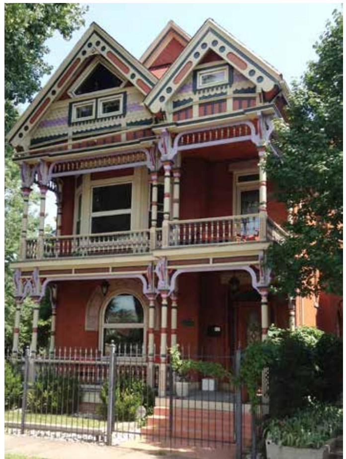
4. High-style Queen Anne on Bryant St. Note the two-story porch with spindle columns and balustrade, fretwork, the forward facing eave with decorative barge-boards, and fish scale shingles
