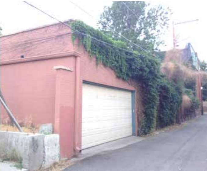
7. Carriage house structures within Clements Historic District. Accessed from the alleyway, one-story in height and of brick construction with a flat roof.
