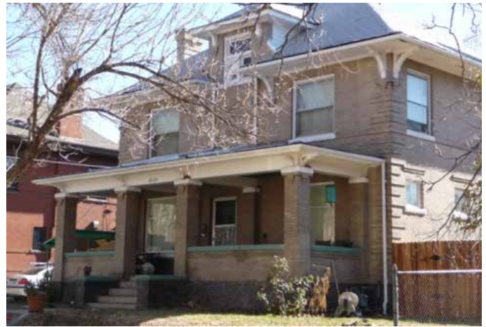
4. Craftsman Denver Square. Note the more decorative features and details, including front dormer window, broad overhanging roof eaves supported by brackets, corner brick quoins, and corbelled masonry piers supporting a full-width bracketed porch.
