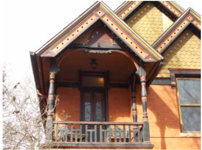
7. Second-story porch detail of a Queen Anne style building. Note the spindle columns, decorative balustrade, ornate barge boards, and the decorative fish scale shingles and sunburst motif in the forward facing eave. Also note the wood panel door with large decorative lights and transom.
