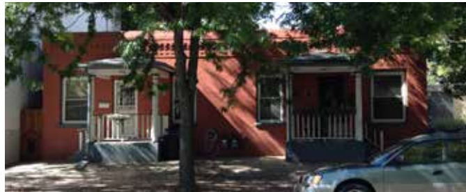
5. One-story Italianate rowhouse with two separate entries. Note the decorative cornice, low hipped porch roofs, stone sills, and absent front yard.
