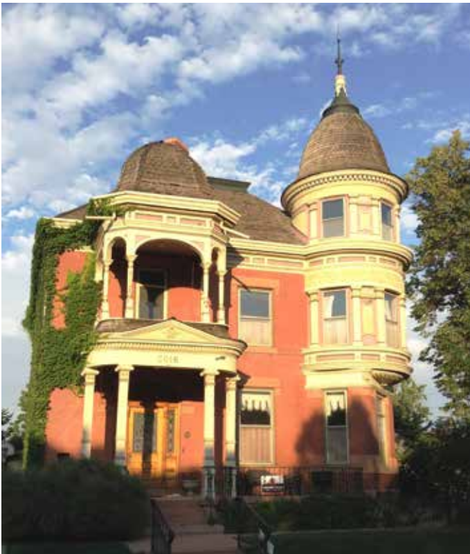
5. High-style Queen Anne located on a corner lot. Note the two-story entry porch with pediment roof line on the first floor and a modified mansard roof on the second floor, the projecting oriel window tower with conical roof and decorative wood elements.
