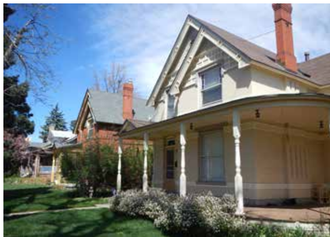
2. Streetscape with Queen Anne style structures. Note the uniform front yard setback, the projecting front porches, and architectural harmony of this block.
