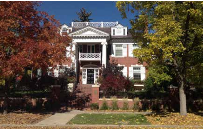
7. The Classic Revival style structure with a large central walkway to the portico entry is typical. Note the historic fenced in front yard with masonry foundation, concrete coping, and iron fence above.
