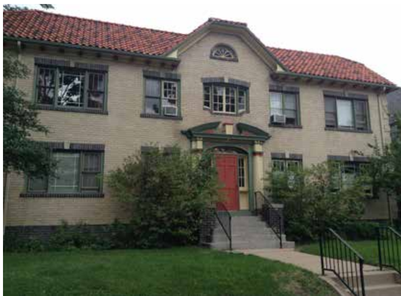
3. Early 20th-century apartment buildings are two to four stories high and are typically designed with an Eclectic or Classical Revival vocabulary. Many have raised foundations and barrel tile clay roofs, such as this one.
