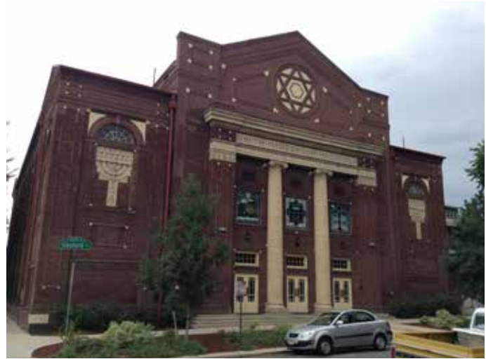
10. Beth HaMedrosh Hagodol was a Jewish synagogue in the Classical Revival Style that has been converted to a Christian church. Note the building's symmetrical massing, prominent entrance, brick façade and terra-cotta ornament.
