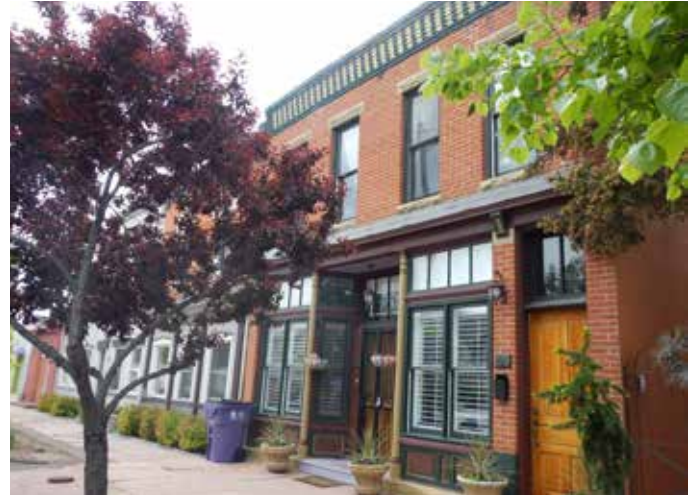
4. Historic commercial development within Baker. Note the two story massing, the recessed central entry with offset side entry, the storefront windows with transoms above and the decorative cornice.
