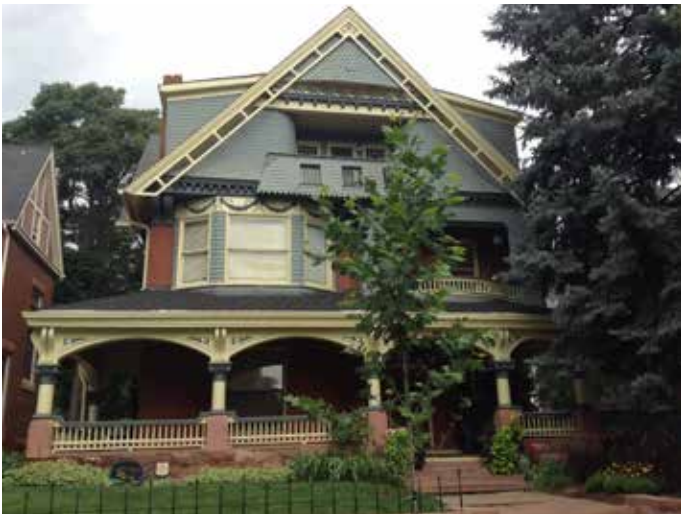
5. The elaborate shingles covering the façade, the arched colonnade at the porch, the decorative bargeboards, and the bay window represent the divergence from the typical Queen Anne style to the Shingle Style.
