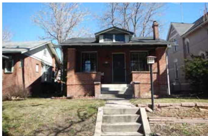
10. Bungalow with a full-width porch under the main roof, and a multi-light dormer. Note the central steps and walkway leading in a straight path to the front entry.
