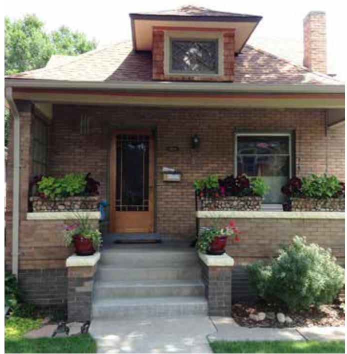
6. Craftsman Bungalow. Note the dormer window in the hipped roof, the masonry porch foundation and piers, the differentiation in brick from the foundation to the primary wall, and the offset entryway.
