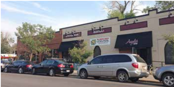
3. Several early 20th century commercial buildings are located on the south side of 6th Avenue with boxy, symmetrical massing.
