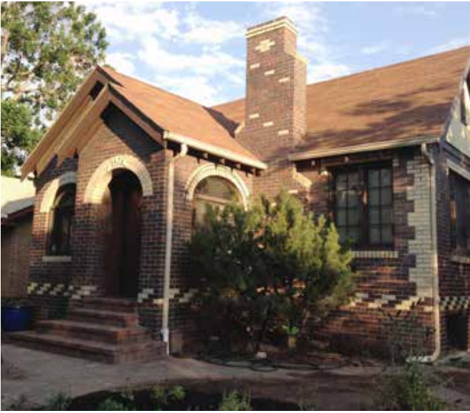
5. Tudor style structure. Note the decorative chimney, the arched porch and window elements, and the multi-divided light windows.
