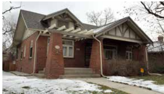
8. Bungalow with a projecting front gabled and trellised full-width porch. Note the half-timbered detailing in the front gable and the battered brick porch columns.
