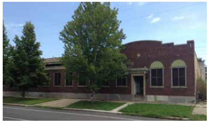
5. Typical early 20th-century commercial development within the district, featuring brick construction and raised parapet hiding a flat roof.
