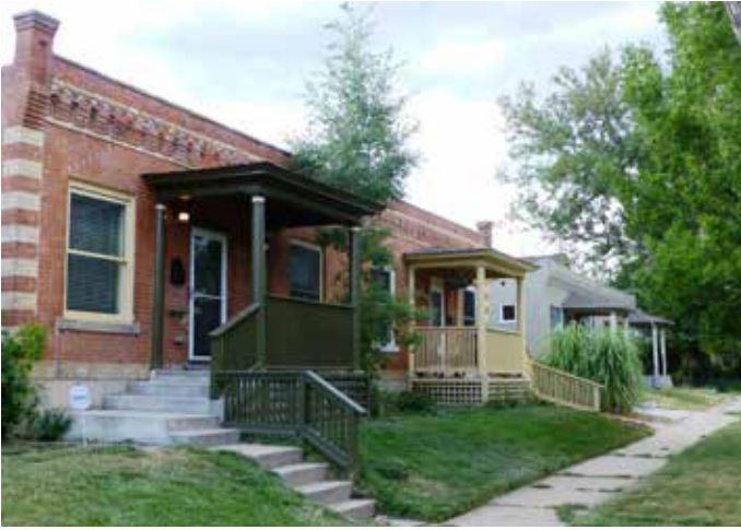
5. Red brick rowhouse with corbelled roof detailing and raised columns at roof parapet. Note steps leading from the sidewalk into the front lawn to accommodate the Denver Hill.
