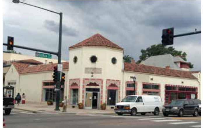
8. Commercial development on Colfax in the Spanish Revival Style. It is one-story high, has symmetrical massing, large display windows with transoms, and a barrel clay tile roof.
