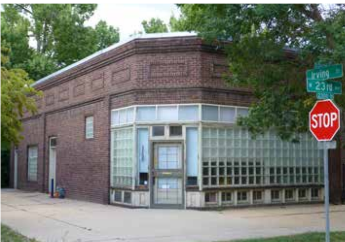
7. One-story red brick commercial building with decorative raised roof parapet located on the 23rd Avenue streetcar line.
