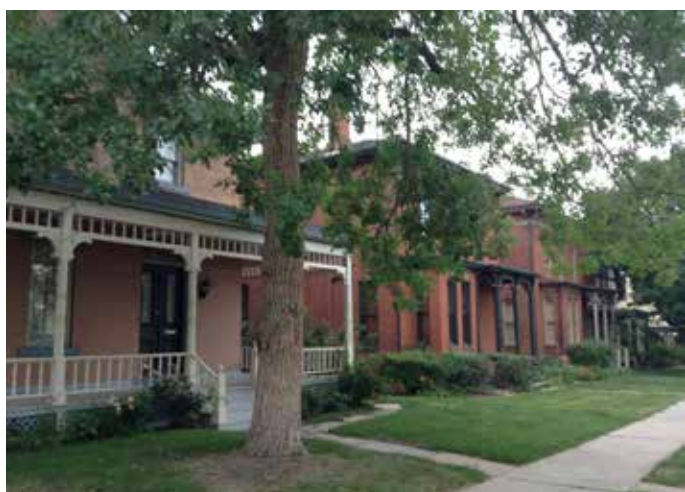
1. Tremont Pl. streetscape. Note the uniformity in the front yard setback, the brick buildings, and projecting front porches of these Italianate style structures.
