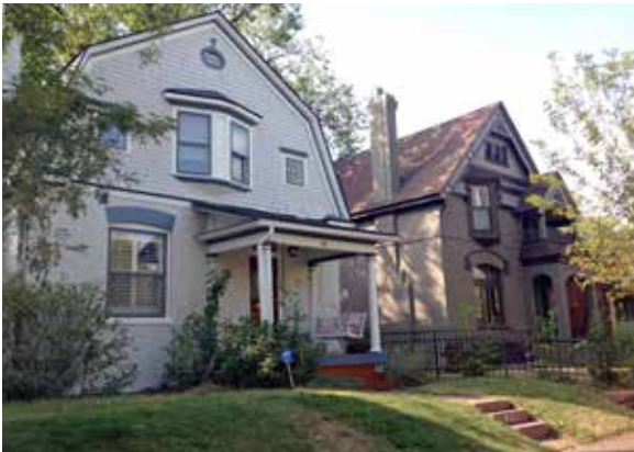
6. Dutch Colonial Revival and Queen Anne style dwellings. Both houses have offset entries with projecting one-story porches, and tall chimneys.
