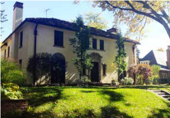
4. This Mediterranean Revival style structure has a stucco façade, a low-pitched barrel tile clay roof, and a central entry with decorative pediment, symmetrical window bays, and multiple chimneys.
