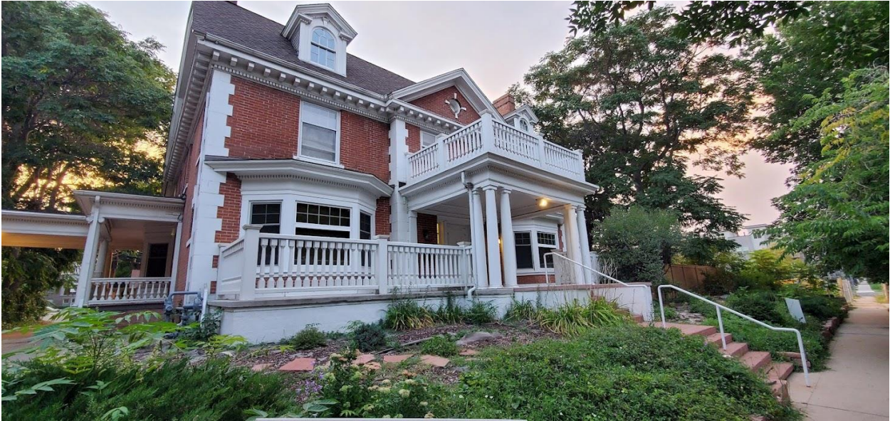
Street level, east side.
