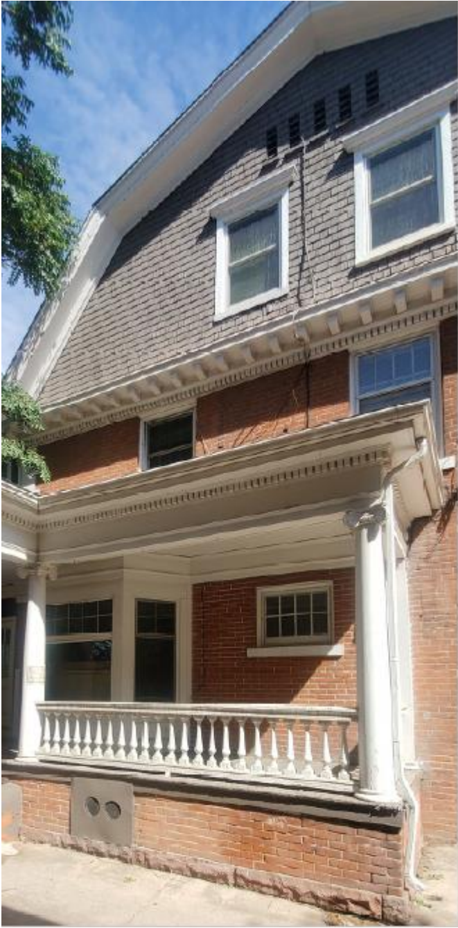
South side showing porch alongside driveway.
