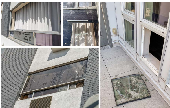
Observations included cracks and other exterior damage, above, and damaged or broken windows, right.
