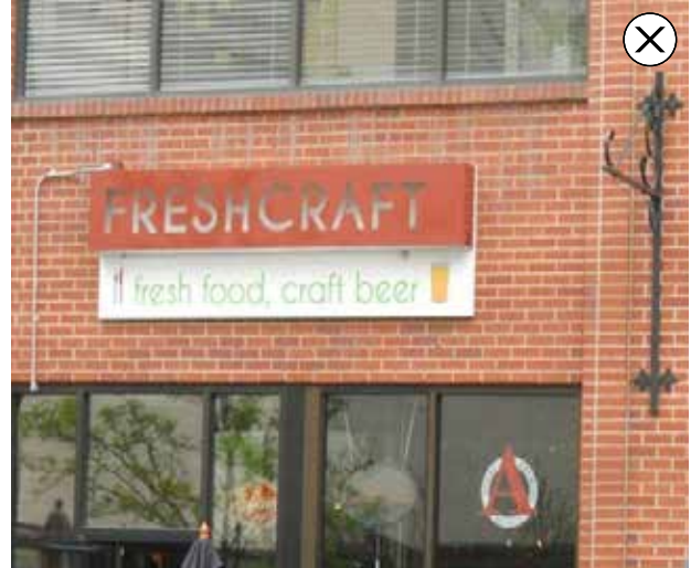
163. Remove remnants of old signage that will not be reused, such as the unused sign bracket in the upper right of this photo, and do not run exposed conduit on the exterior of the building.
