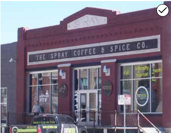
168. When using an existing sign band, provide space between the sign and the sign band edge. Keep sign flush with painted or pin mounted letters.
