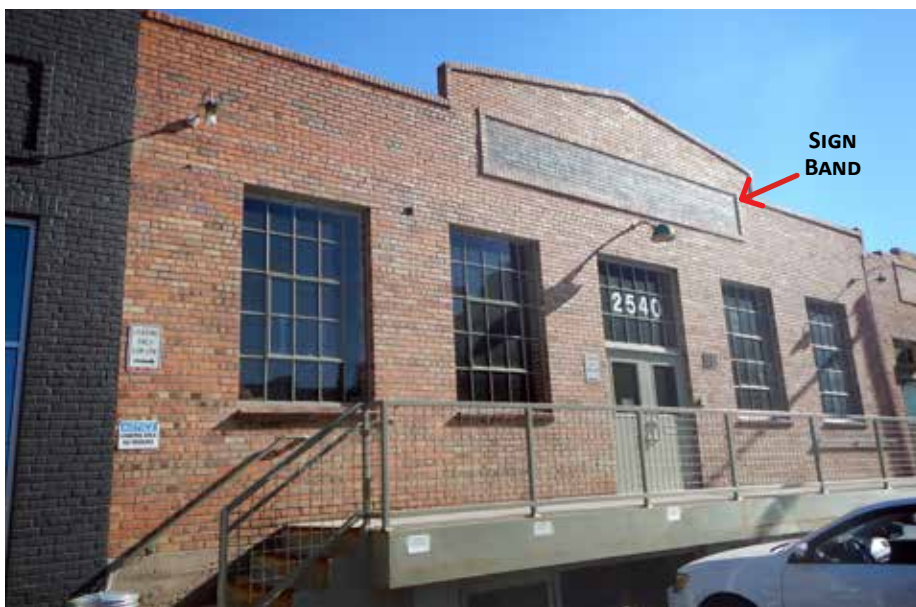
150. This building has an original sign band centered over the front door which would be a good signage location for a future user.
