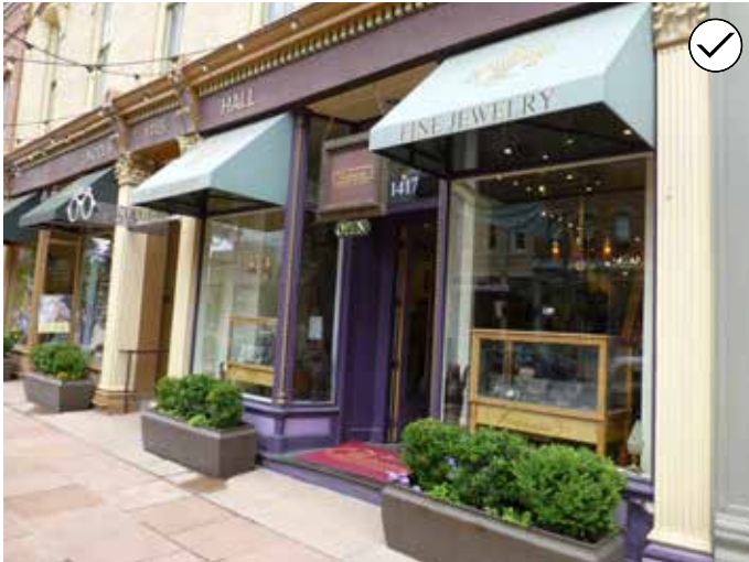
156. Coordinate sign locations, types and sizes to create consistency among multiple tenants in one building, such as the multiple retail tenants in this building.
