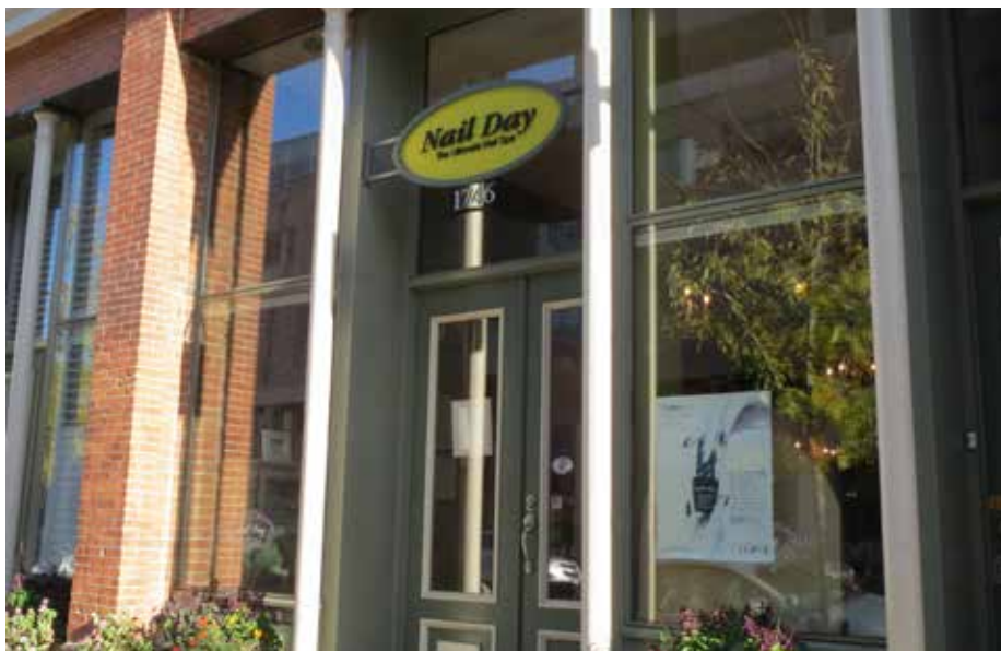
149. This signage was installed to limit impacts to character defining features of the building, such as the cast iron columns.
