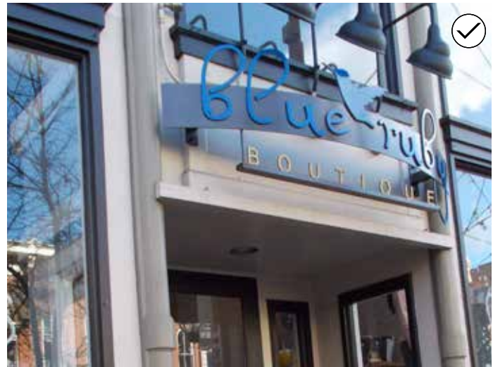
169. A slightly arched sign can still be considered a wall sign if it extends off the wall plane by 2 feet or less. This wall sign does not obstruct architectural details of the building.
