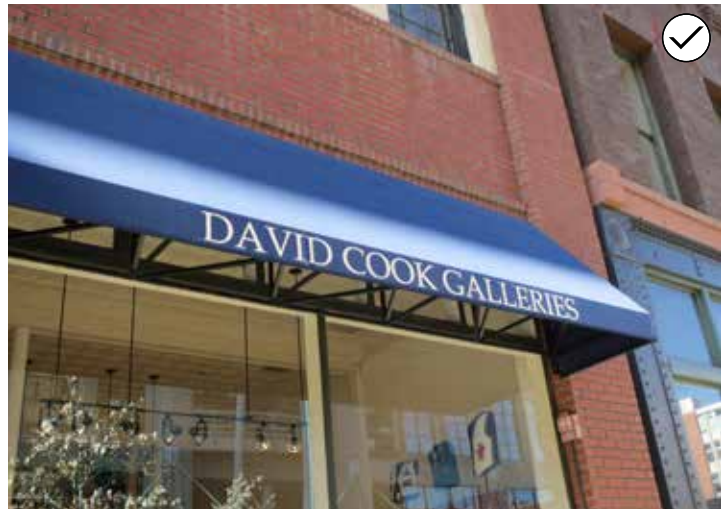
173. Use traditional triangular shaped awnings comprised of high quality canvas to frame a storefront window or door.
