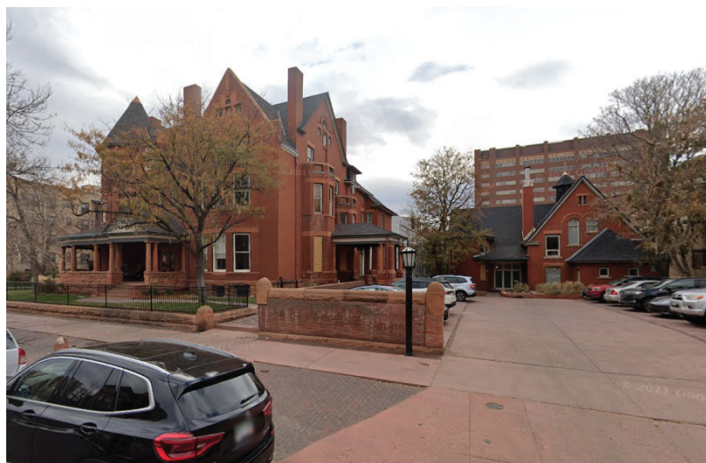
Today, the Grant Street Mansion is listed in the National Register of Historic Places. Source: Google Streetview
