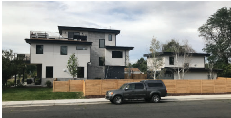
An example of a primary house and ADU on a 6,270 sq ft lot in the E-SU-D1x zone district. Source: CPD
