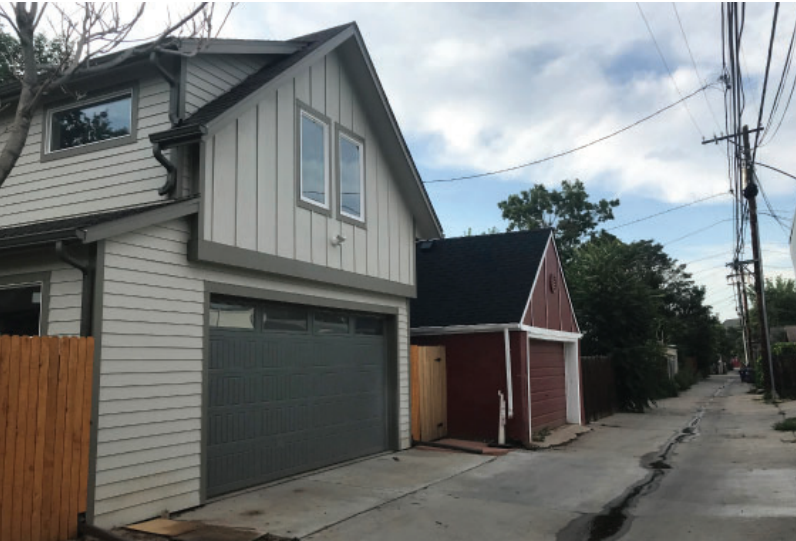
An example of an alley improvement due to ADU development. Source: CPD
