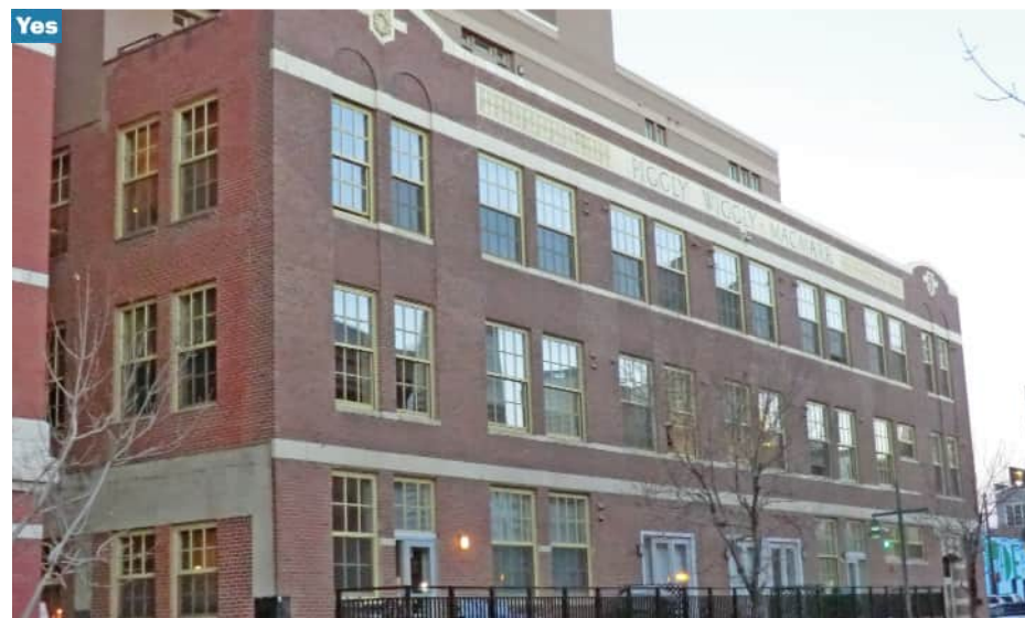
Left: Locate an addition to be subordinate to the original structure, such as this commercial rooftop addition that is setback from the primary facade.
