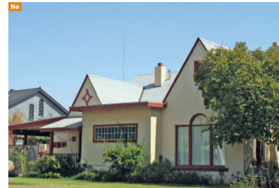
Left: Remove a non-historic addition that detracts from the historic appearance, such as this front facade flat roof addition.
