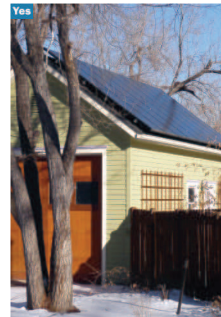
Left: Solar panels may be installed anywhere on the roof of an accessory structure. Middle: Solar panels placed on an unobtrusive location on the rear roof slope. Right: Solar panels should be installed at least 3 feet back from the diagonal roof ridge to reduce visual impact. These panels are not set back 3 feet.
