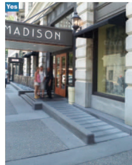
Left: An exterior ramp at the primary building entry, ensuring that it is easy to find. Middle: A ramp integrated into the historic loading dock. Right: A ramp integrated into the landscape setting.
