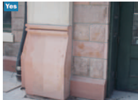
Top Right: Do not allow an original foundation to fall into disrepair. Left: A damaged pink sandstone foundation. Middle: The damaged sandstone foundation was patched with a consolidant that was tinted to match the existing pink sandstone.
