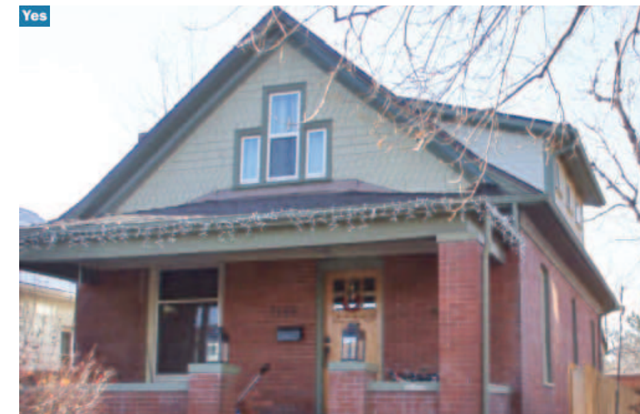
Left: Design a dormer to be subordinate to the overall roof mass and scale with those on similar historic structures. The dormer is set back behind the overhanging roof eave and adjacent brick wall plane.
