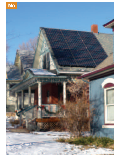
Left: Solar panels may be installed anywhere on the roof of an accessory structure. Middle: Solar panels placed on an unobtrusive location on the rear roof slope. Right: Solar panels should be installed at least 3 feet back from the diagonal roof ridge to reduce visual impact. These panels are not set back 3 feet.
