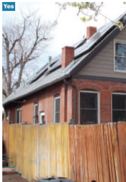
Left: Solar panels placed to avoid chimneys. Right: Solar panels placed flush to the roof surface and around cross gable roof form.
