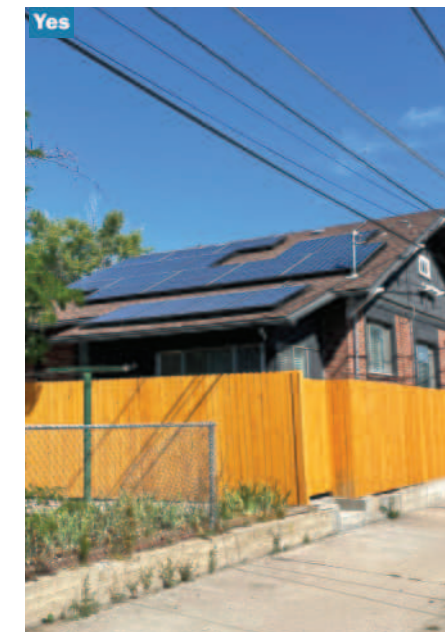
Left: Solar panels may be installed anywhere on the roof of an accessory structure. Middle: Solar panels placed on an unobtrusive location on the rear roof slope. Right: Solar panels should be installed at least 3 feet back from the diagonal roof ridge to reduce visual impact. These panels are not set back 3 feet.
