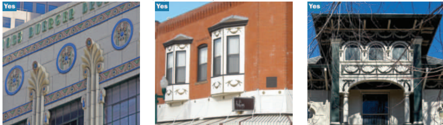
Left: Retain and treat exterior stylistic features and examples of skilled craftwork, such as these terra cotta columns and art deco medallions with sensitivity. Middle: Preserve significant stylistic and architectural features, such as bay windows and masonry detailing. Right: Preserve significant stylistic and architectural features, such as decorative ornament, brackets, trim and moldings.
