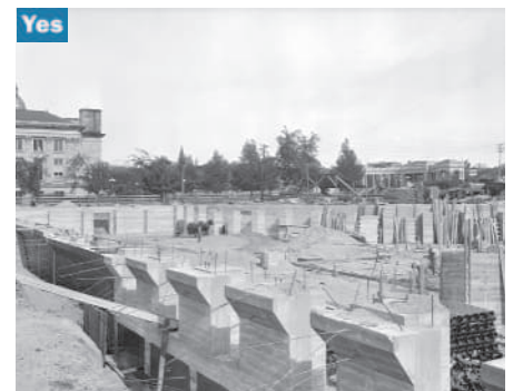
Right: 1929 construction photo of the Denver City and County Building, DPL Digital Collections, call no. X-27518
