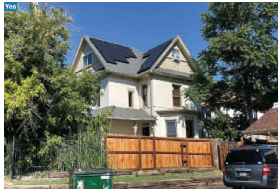
Left: Solar panels placed to avoid chimneys. Right: Solar panels placed flush to the roof surface and around cross gable roof form.
