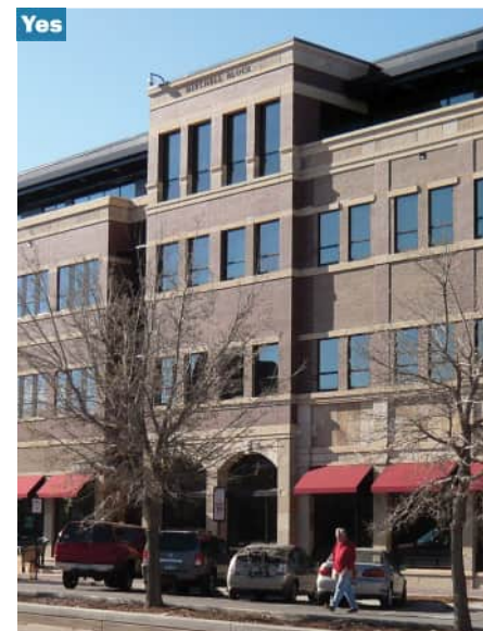
Top Right: Use materials that help to convey scale in their proportion, detail and form. Bottom Right: Use vertical and horizontal articulation design techniques to reduce the apparent scale of a larger building mass.
