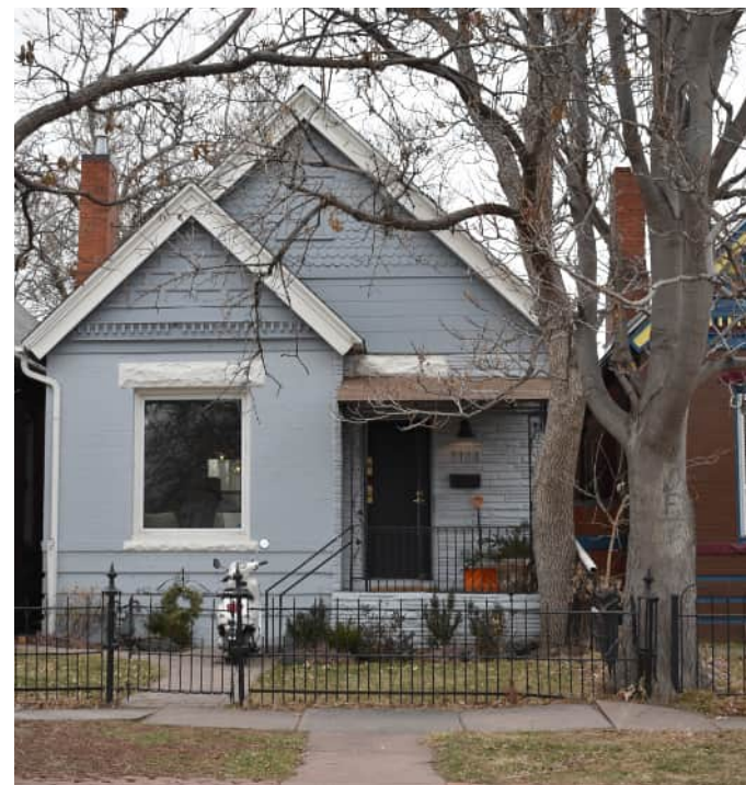
Left: A contributing structure in La Alma Lincoln Park with perma-stone around the porch and earlier decorative trim in the gable faces.
