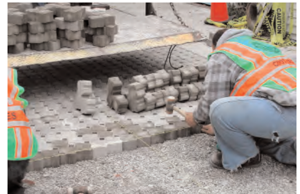
Permeable pavers in parking lots (above) and alleys (below)
