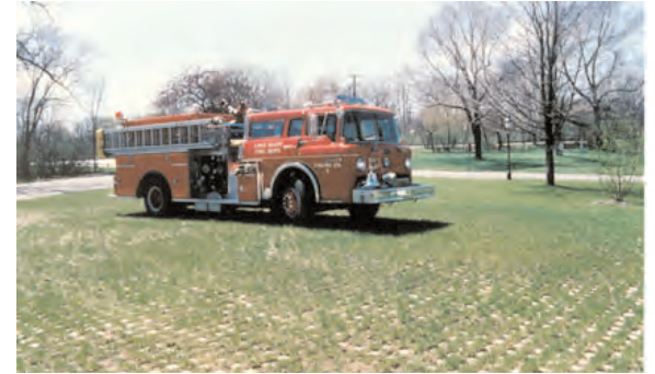
Permeable pavers in parking lots (above) and alleys (below)
