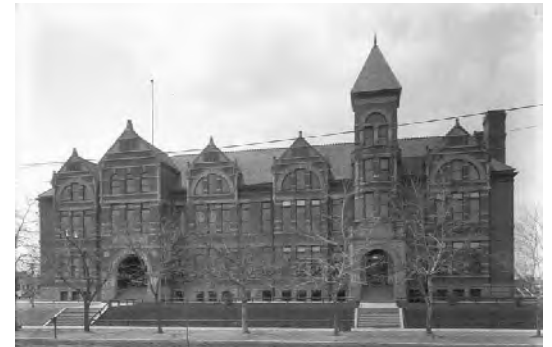
Historic Cheltenham School, demolished in the 1970's for "urban renewal".
